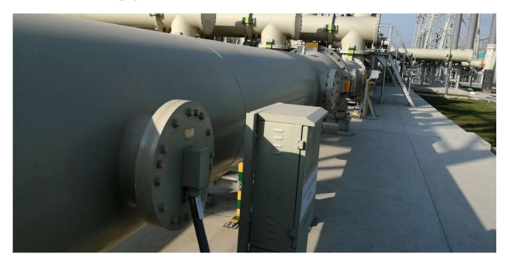
GIS ( Gas Insulated Switchgear ) degradation might lead to complete GIS breakdowns. PDGuard-G5000 detects and alerts various defects inside of GIS by analyzing UHF signals generated by partial discharge . It's easy to deploy for permanent or shorter term monitoring and highly cost-effective .
